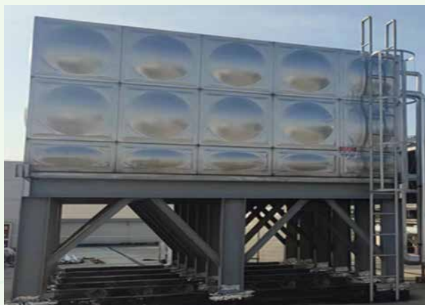
Suzhou Factory's condensate and rainwater recovery systems
